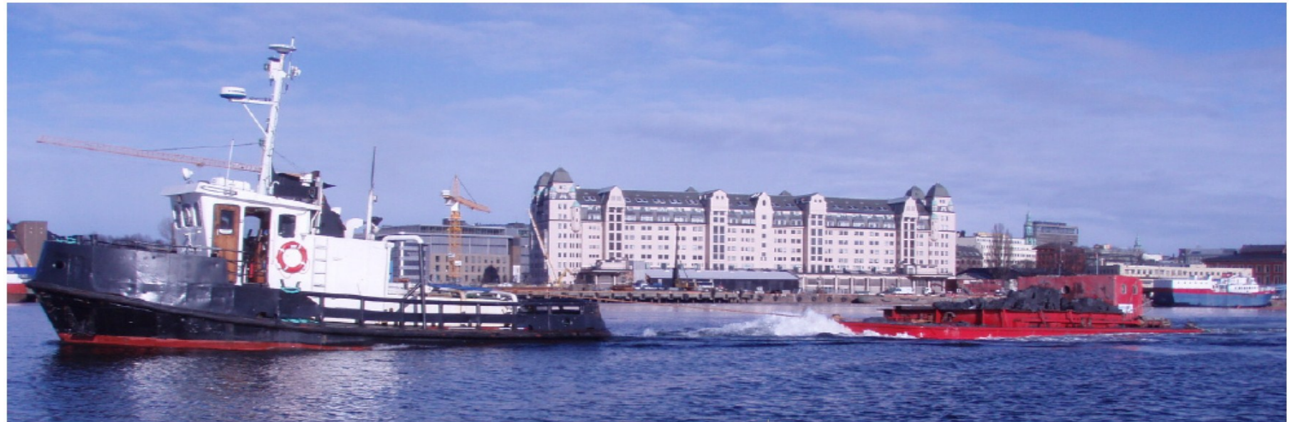
Remediation project of Oslo harbour.
